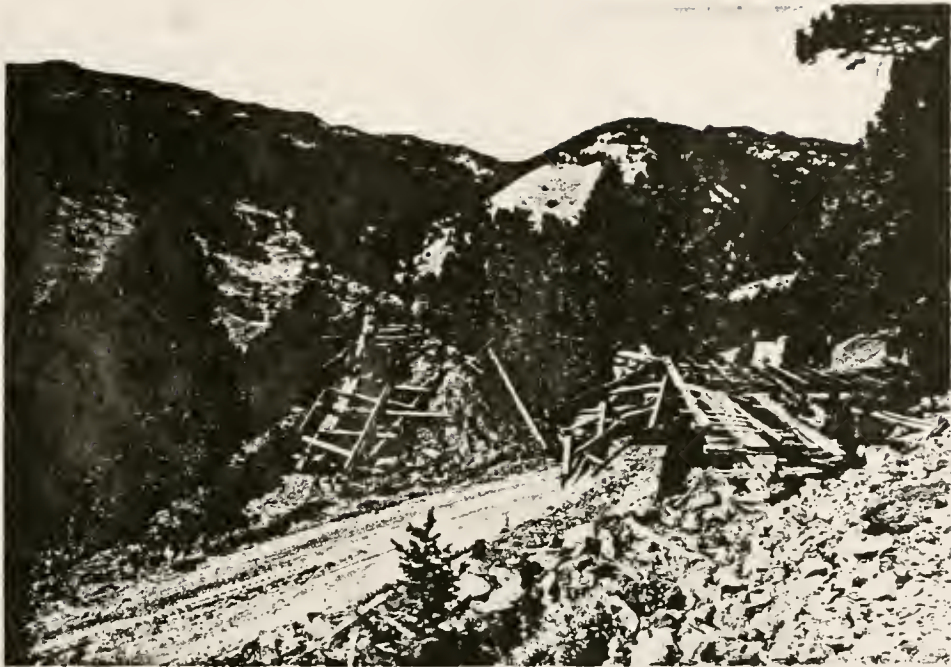
Figure 231. Feature #115 (trestle), northwest view.
